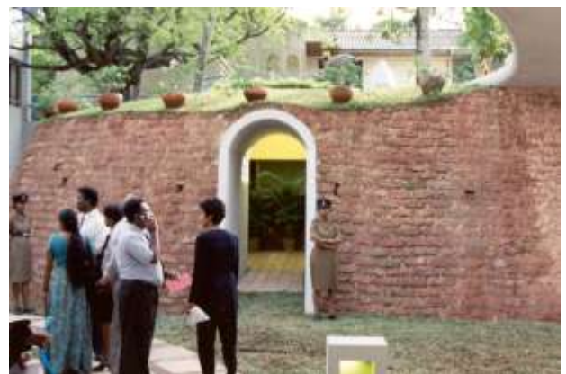
Most of the original site landscape was kept - here an earth berm with huge trees on top. It was cut through to access a part of the building. Note that yellow is used wherever a lightshaft occurs to let daylight into interior spaces to save on use of electric light.
