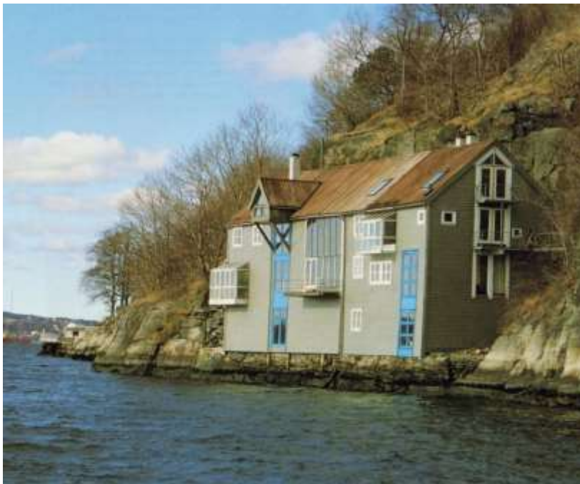
Traditional wooden building in Norway: Old fish warehouse in Bergen, converted to housing, with heat pump, passive solar, etc. Architects Butters / Bruskeland / Haukeland
