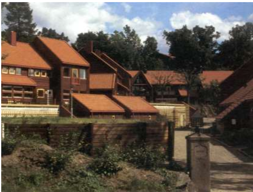
Low dense cluster housing in timber, Oslo Giskehagen, Torp architects
