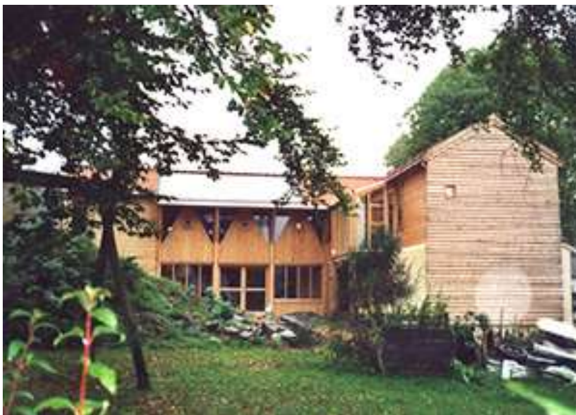
Timber low energy house, Stavanger Architects GAIA Lista
